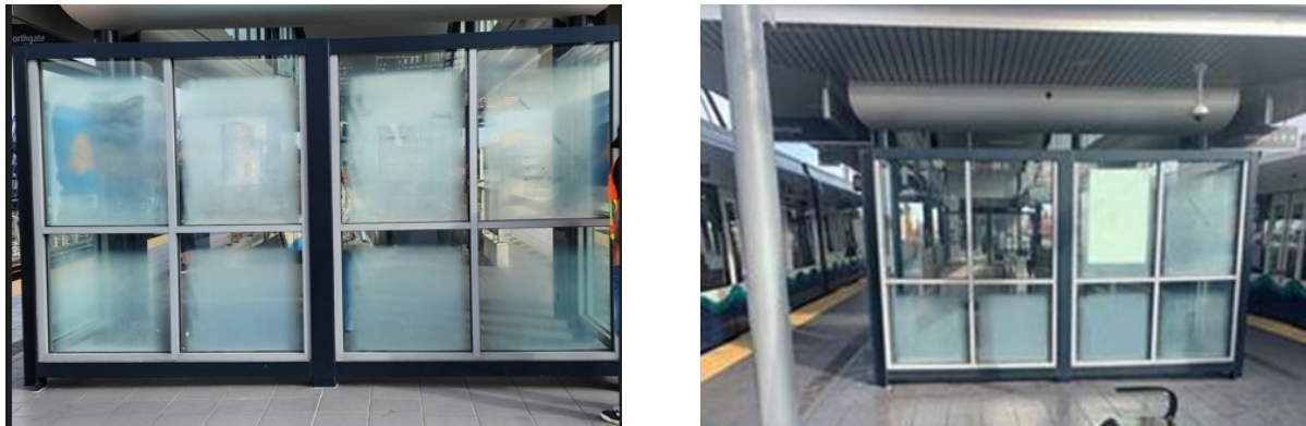
Figure 15. Before and during replacement of anti-graffiti film at Angle Lake Station
